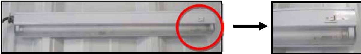
Wall-mounted florescent with shield over entire bulb ideal for lighting on dark walls or syrup grading
